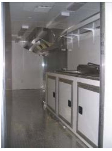
Inside picture of the trailer featuring the built in sinks and the commercial exhaust hood that will house the ovens, range and tilt kettles. Water storage tanks and heater are under the counter.
